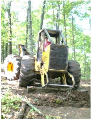
The first push on a water bar should extend beyond the upper edge of the skid trail. The skidder should be articulated to provide the correct 30 degree angle for the water bar. The skidder should pull up to within 2-3 feet of the correct location for the waterbar. To start construction, put down pressure on the skidder blade, lifting the front wheels off the ground. Ease the skidder forward 2-3 feet to create the waterbar.
